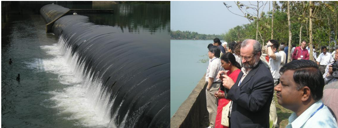
Photo 7: Left: rubber dam, right: visitors to the rubber-dam project
